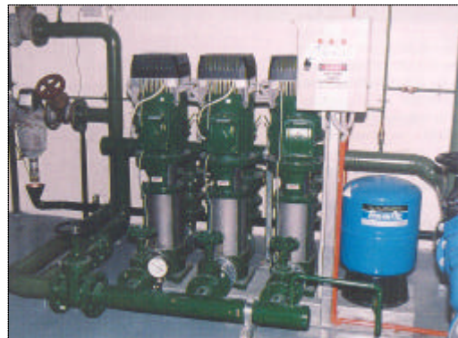
Kelair's Packaged Variable-Speed-Drive and Fixed-Speed-Drive Pressure Systems designed to draw water from tanks, dams, rivers and direct connection to town's main to provide flow and pressure requirements by conventional system or one operating as a variable speed drive unit.
